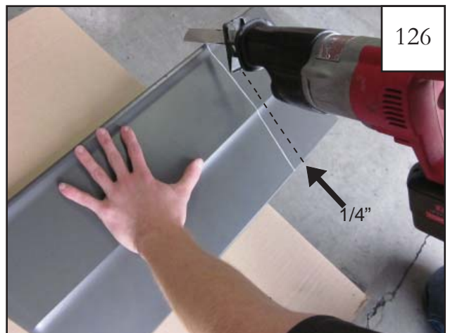
Using a reciprocating saw or other suitable tool, cut the factory side cladding approximately 1/4" back from the line drawn in step 122.
