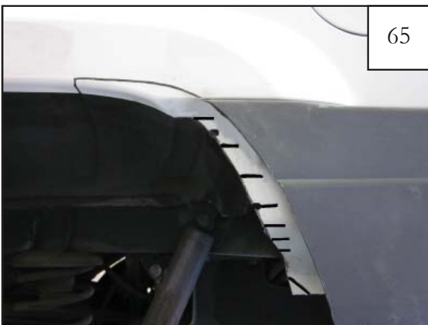
Mark vehicle for cutting: Make lines on sheet metal as shown in picture.
