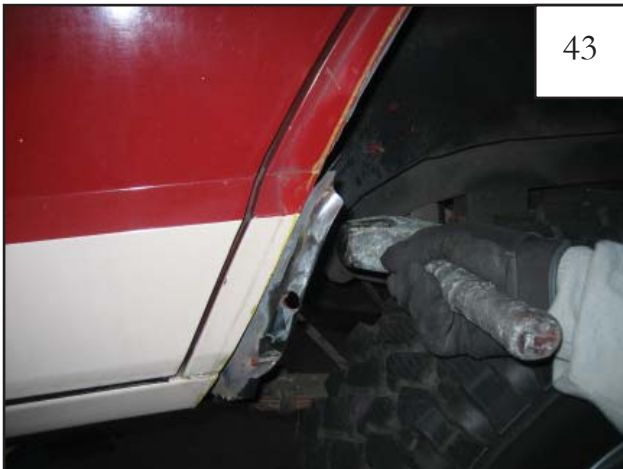
Using a hammer or mallet, pound the inner sheet metal layer over the seam.
