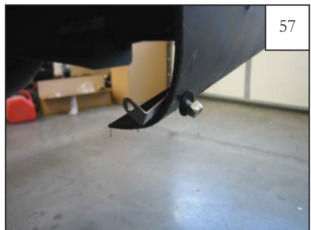
Start a washer, screw, and nut combination through the two holes and brackets in the bumper.
