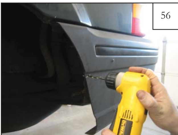
Using a 3/16" drill bit, drill the two marks made in step 55.
