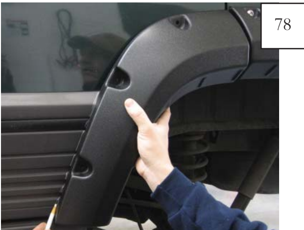
78 Close rear door. Hold door piece in place on door aligning it with rear main flare and trace outer edge of flare onto body side molding. Part is marked on the inside. Driver's side: LR3 for door piece.
